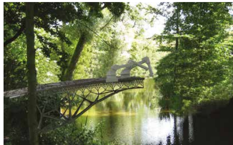
Right: A 3D printer with robotic arms building a pedestrian bridge in the Netherlands (© MX3D Joris Laarman Lab)
